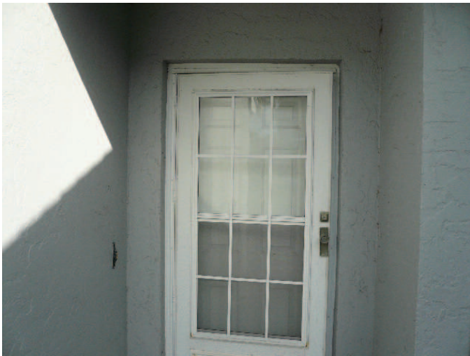
Not shuttered or labeled as impact rated
