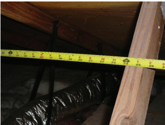
24" truss spacing
