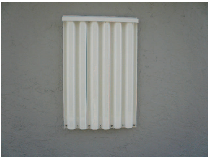
Large missile impact rated shutters
