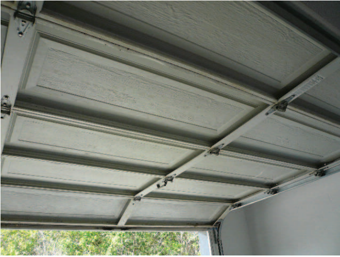
Not shuttered or labeled as impact rated
