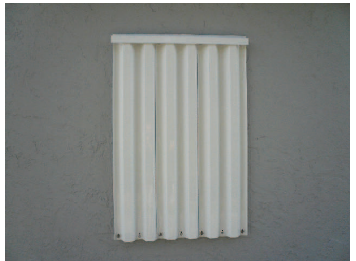
Large missile impact rated shutters
