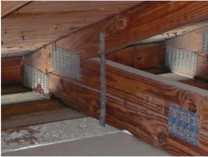
Strap with 5 nails / Does not wrap over truss
