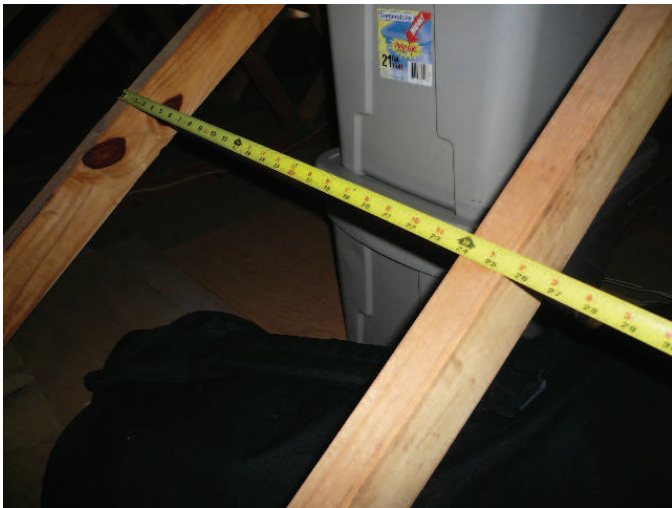
24" truss spacing
