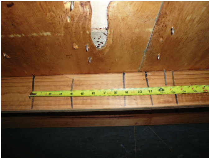
8d nails on 6" spacing
