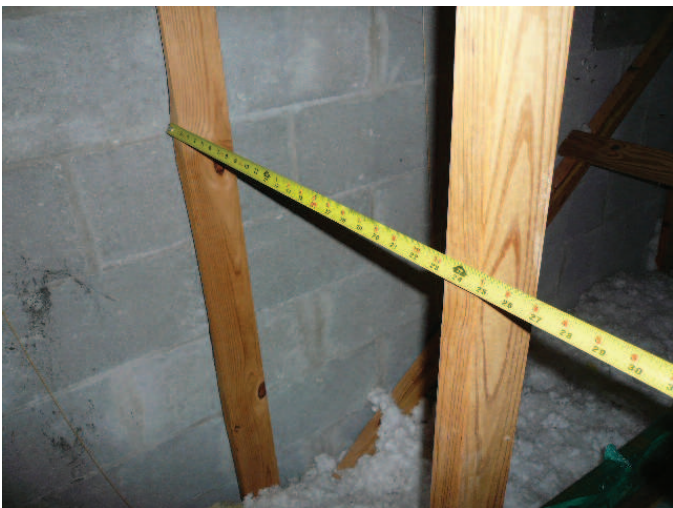
24" truss spacing
