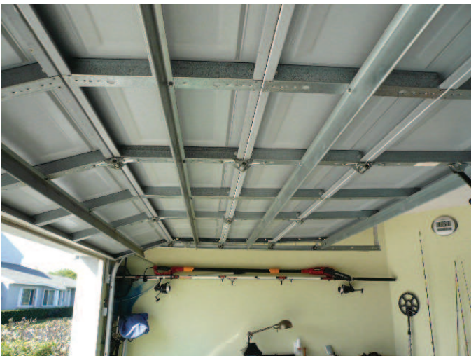
Not shuttered or labeled as impact rated
