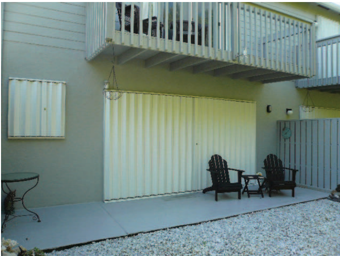
Non verified shutters
