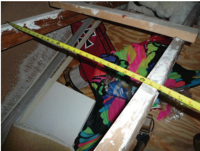
24" truss spacing
