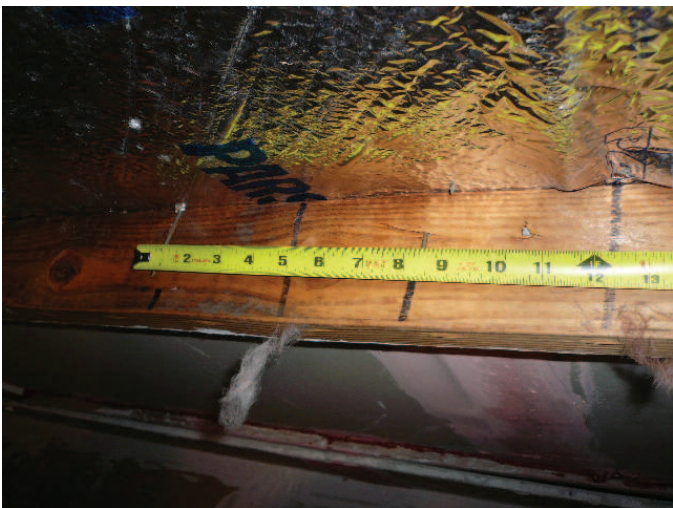
8d nails on 6" spacing
