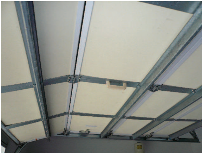
Not shuttered or labeled as impact rated
