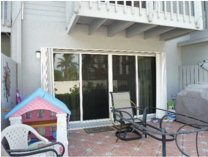
Non verified shutters
