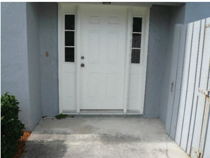
Non verified shutters
